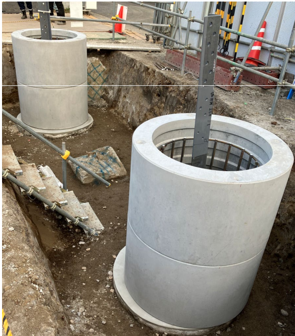
Figure 5: Photos of Precast Foundation on Construction Site
