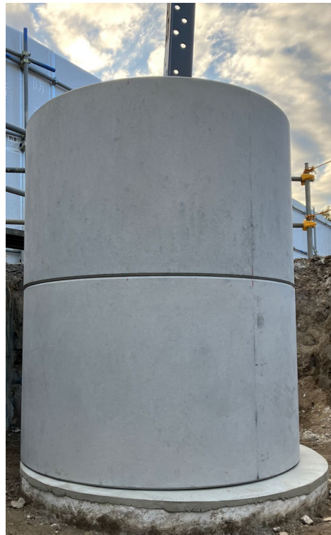
Figure 5: Photos of Precast Foundation on Construction Site
