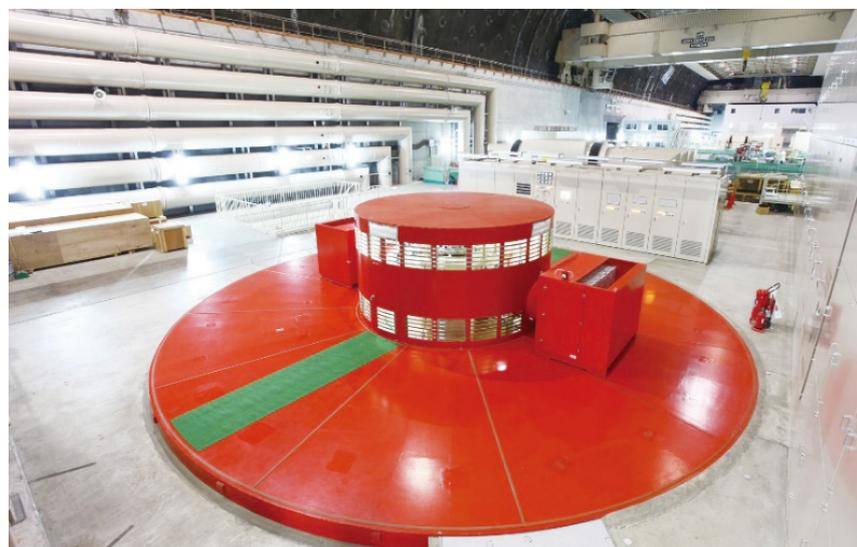
The large-scale Adjustable Speed Pumped Storage Power Generator commenced in 2014 (Generator No.4 at TEPCO's Kazunogawa Pumped Storage Power Station, Japan)
